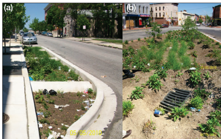
Figure 2. Examples of advanced bio-infiltration projects established in the Baltimore Street subwatershed of WS263. Photos show (a) curb extension with three underground tree boxes and (b) bioretention BMP installations. Total costs for the curb extension installation were over $79 000, including over $16 000 for design. Total costs for the bioretention installation were over $170 000 and included over $38 000 for design.
