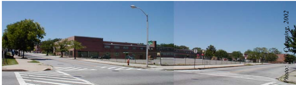
Franklin Square Elementary School
